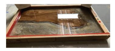
**Tip**: If you're doing multiple pours, wait 2-6 hours before doing another pour. You want to pour the next layer when the epoxy is still in the gel state and the heat caused by the reaction has dissipated. If you wait for the surface to harden completely, you'll need to sand in between pours (using 120 grit, vacuum, & solvent wipe clean). Continue to pour in shallow layers until you reach the desired thickness
